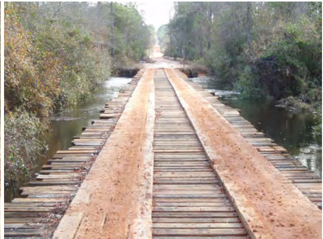
Truck Trail 17 Styx River bridge MP 1.4 (06 February 2010).
