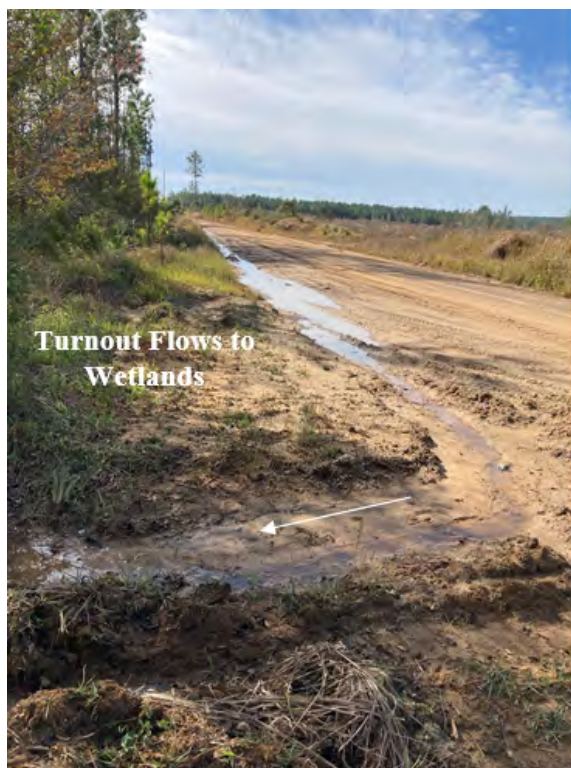
Stormwater Turnout Directed to Wetland
