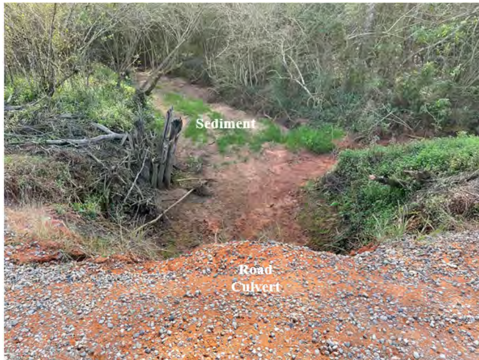
Road Culvert Discharges to Down Stream Wetlands and Stream
