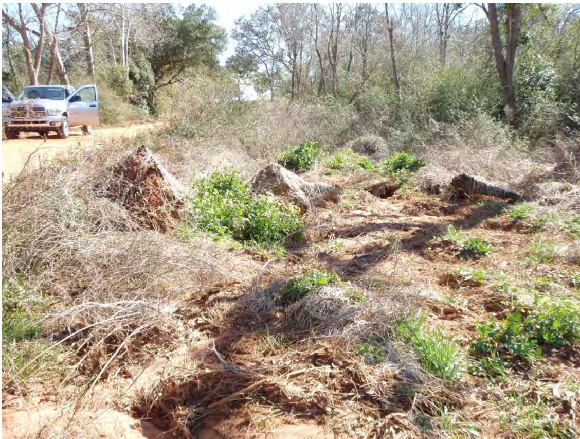
Mannich Lane (S2) near MP 0.3 (20 February 2010).
