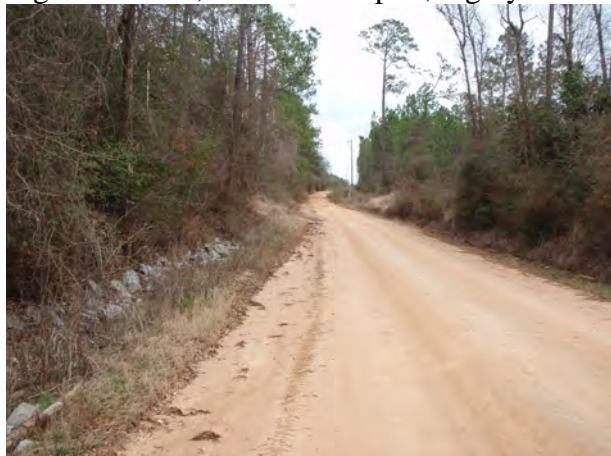
Photo 1: Example of previous ditch line treatment.
