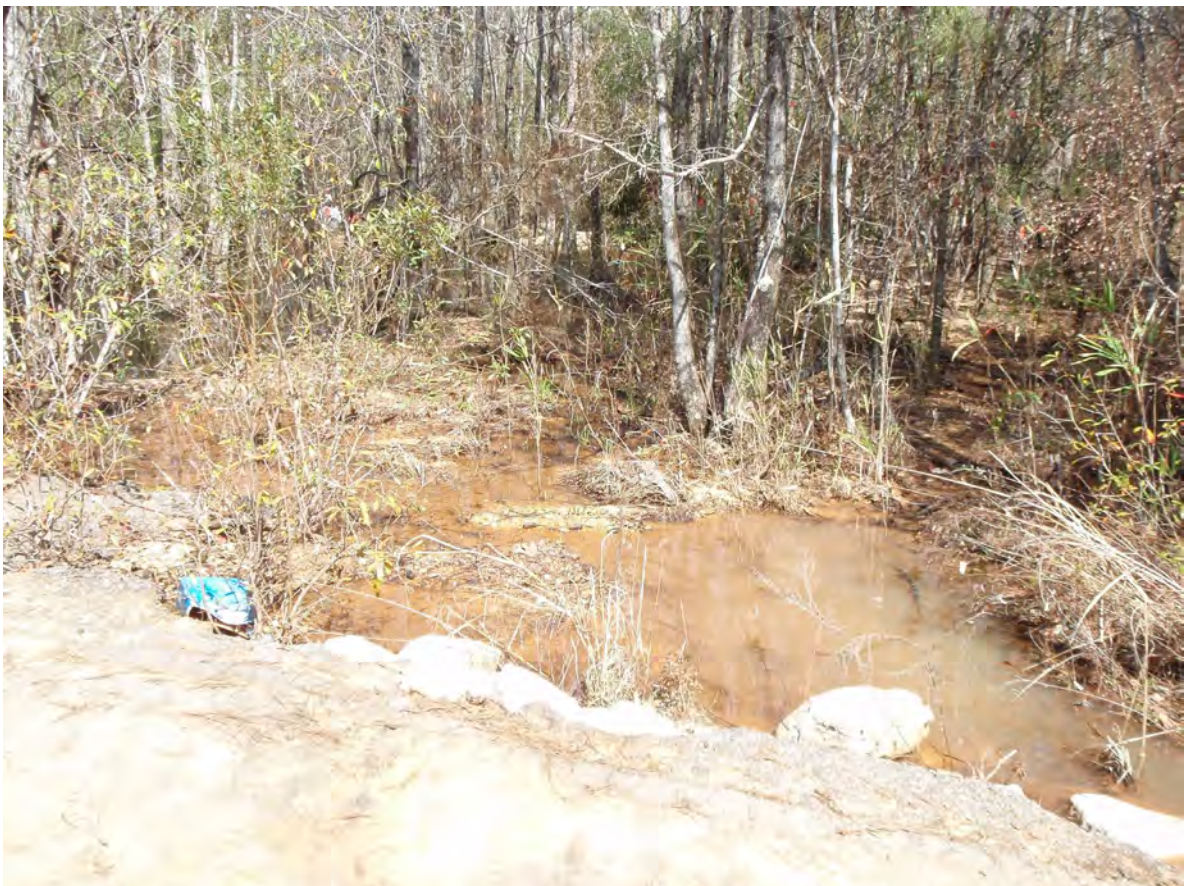
Holly Creek Road sediment impacts to stream and wetland (12 March 2010).
