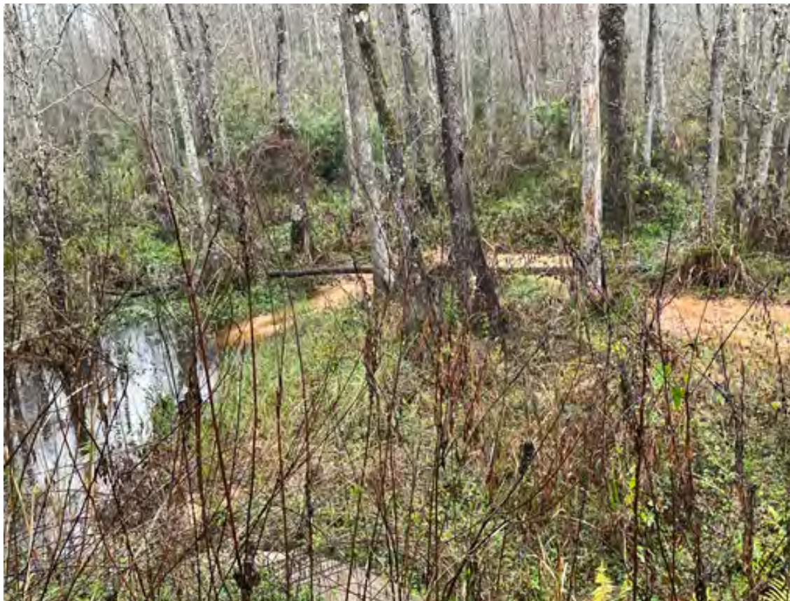
Sediment in Wetlands at Road Culvert
