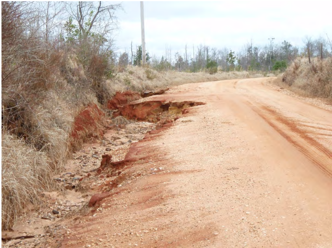
Griggers Road near MP 1.8 (6 February 2010).
