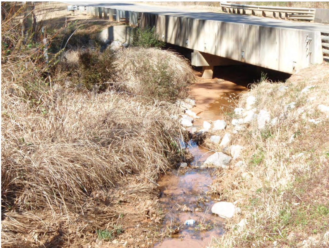
Bretz Lane discharge to Mifflin Creek MP 0.0 (20 February 2010)
