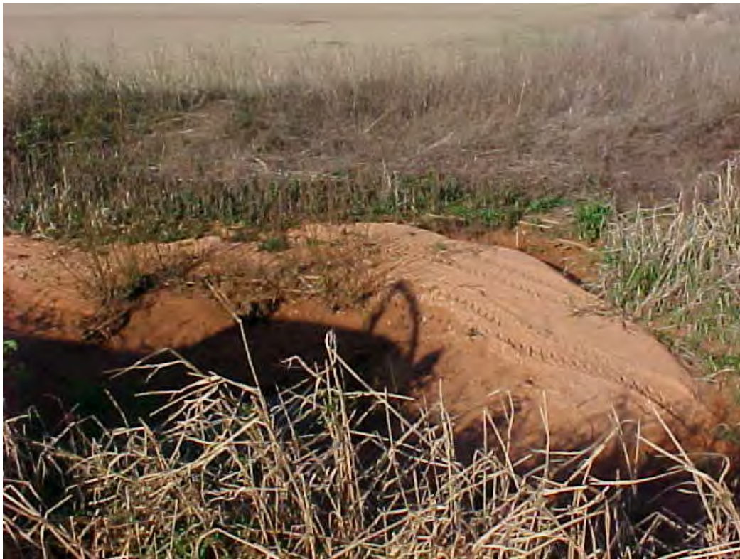
Sherman Road near MP 0.4 (16 March 2010).
