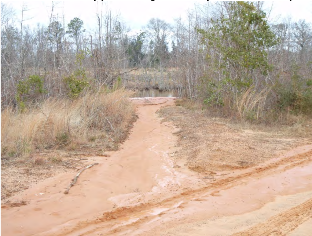
Brady Road near MP 5.0, sediment from turnout impacting Grady pond (6 February 2010).
