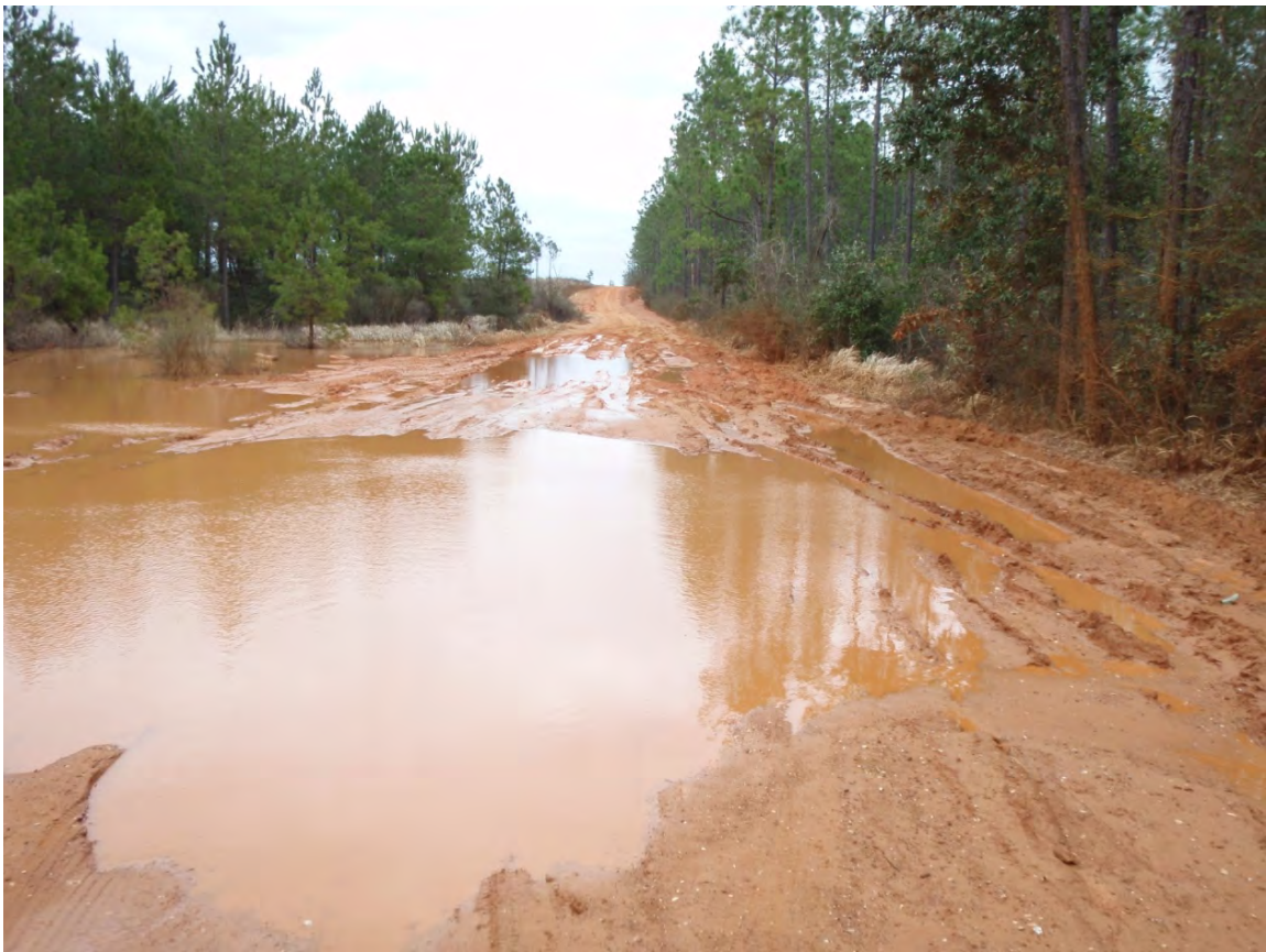
Barrineau Park Road wetland crossing MP 2.2 (6 February 2010).
