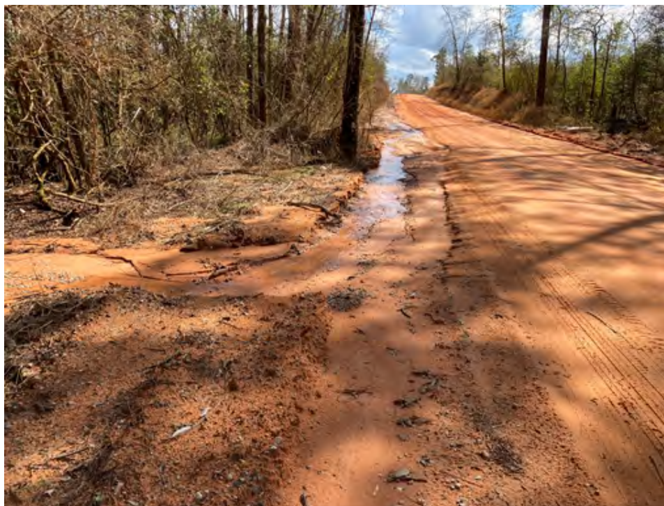
Road Turn Out Directed to Wetlands Adjacent to Hollinger Creek
