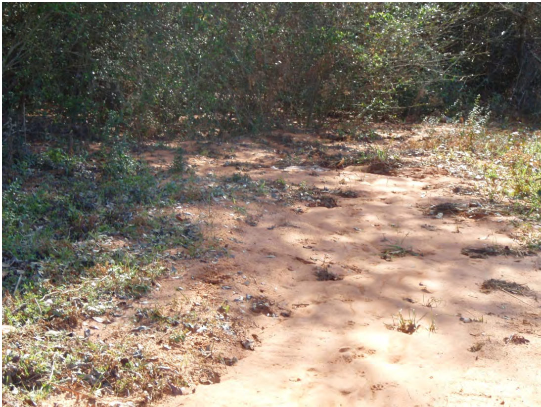
County Road 26 near MP 0.7 (20 February 2010)
