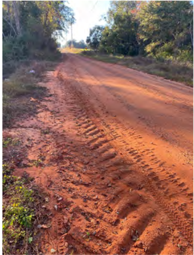
Bay Road East at Creek Crossing
