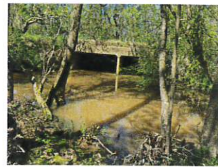
IMG_0395-View North Culvert
