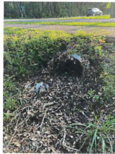
IMG_0542-View Facing West Debris Removed
