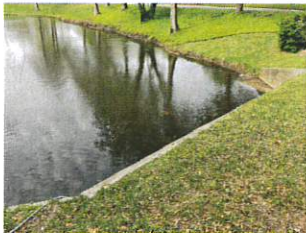
IMG_0577-View Downstream at Pond
