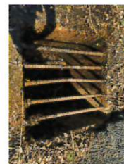
IMG_0412-View Upstream Debris Removed
