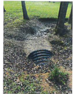
IMG_0539-View Facing South
