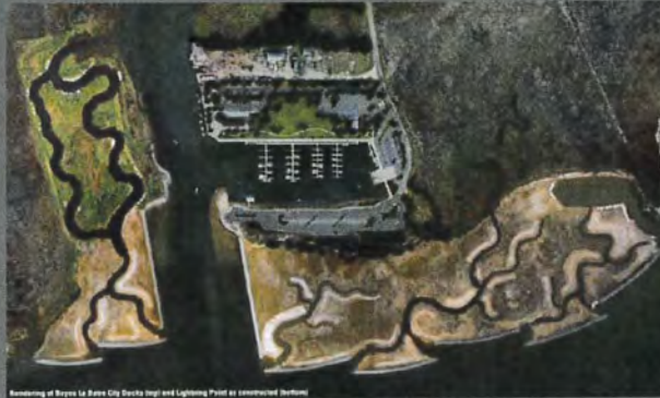
Restoring the Bayou La Batre City Docks and Lightening Point as Constructed Wetland
