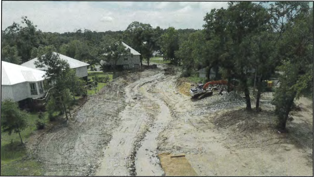
Photo of different phases of project construction.
