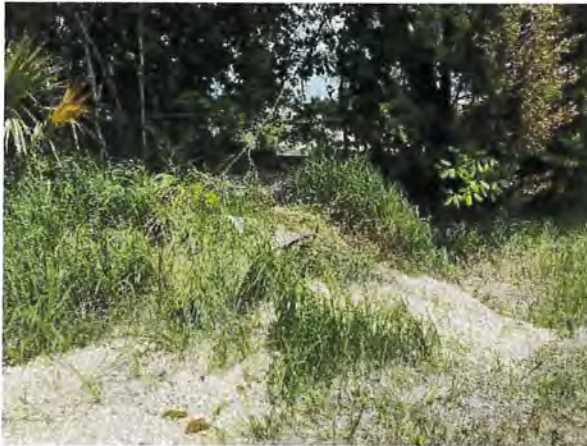
Photo Taken: 6/21/2022 2:18 PM Aggregate and sand discharge offsite.
