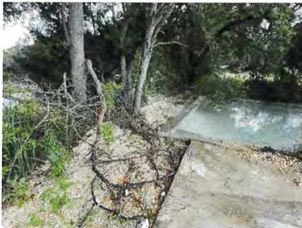
Photo Taken: 6/21/2022 3:34 PM Washout Pit.
