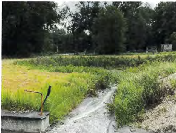
Photo Taken: 6/21/2022 3:35 PM Retention pond.
