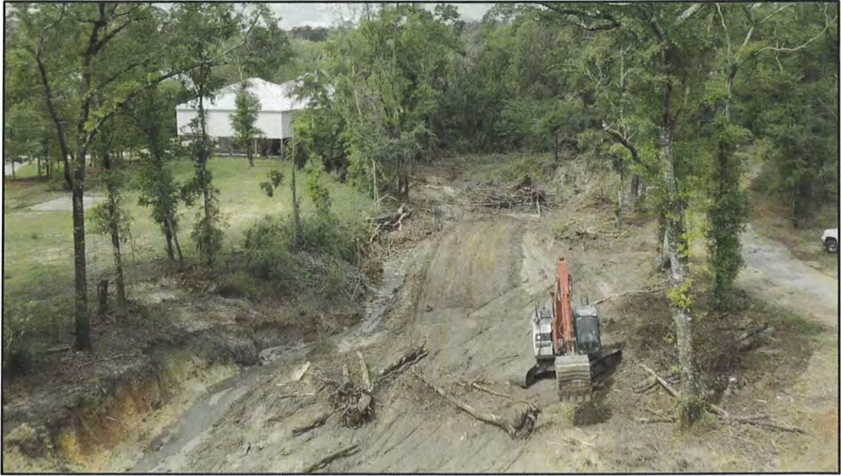
Photo of different phases of project construction.
