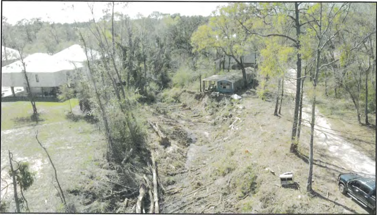
Photo of different phases of project construction.
