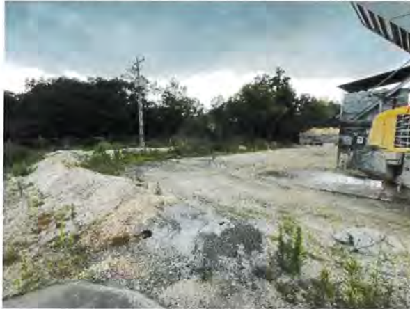
Photo Taken: 6/21/2022 3:27 PM DSN002-1 area with berm.
